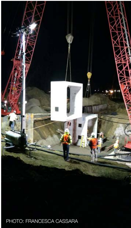
Allen Creek Berm Tunnel installation
